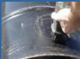
OK, here is where you make your money with your saber saw(sawsall). It does an excellent job of cutting out the round holes for all the vent pipe connections.
