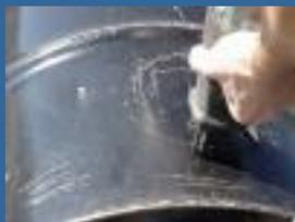
OK, here is where you make your money with your saber saw(sawzall). It does an excellent job of cutting out the round holes for all the vent pipe connections.
