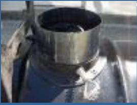
Then I placed the small piece of stove pipe on the damper of the bottom barrel. I used it to hold the top adaptor in place while I marked the holes.
