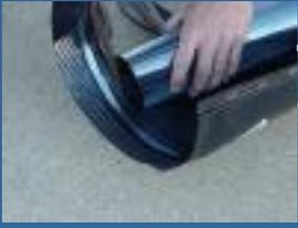
I cut a small piece of stove pipe, about 3 inches. (HINT) To get a close measurement place the top barrel in the seperator legs and hold the collar up to the bottom barrel. This will let you get close to the size of stove pipe.
