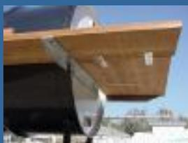
Here is a photo under the shelf. You can see I just tied them together with some zinc plates and screws. You also get a better look at the angle iron I used to hold the shelf on. Notice the notch in the angle iron so it fits up tight on the barrel.
